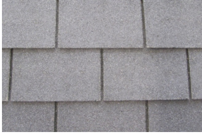
Picture: Three TAB Shingle roof
